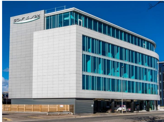
Modern granite cladding – Depending on the context, the use of granite cladding panels in new buildings can work well, as at the GDF Suez building on North Esplanade West.
