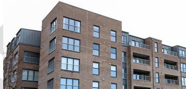
Metal cladding creates a roofscape at Craiginches
