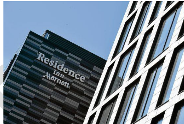
Variations in the colour of panels on the Marriott hotel
