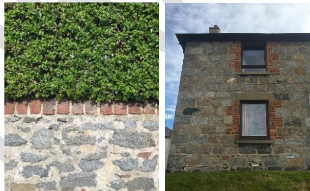
Granite wall with brick coping and window surround detailing – characteristic 'Seaton red'
