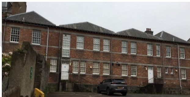
Red brick rear façade of 111 Gallowgate
