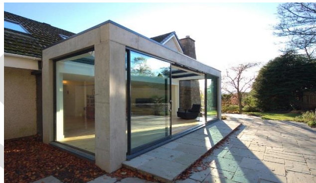
The use of glass in this house extension maximises daylight receipt and minimises the extension's massing
