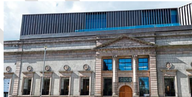
The red/brown colour of the Art Gallery roof extension reflects that of the pink Corrennie granite below.
