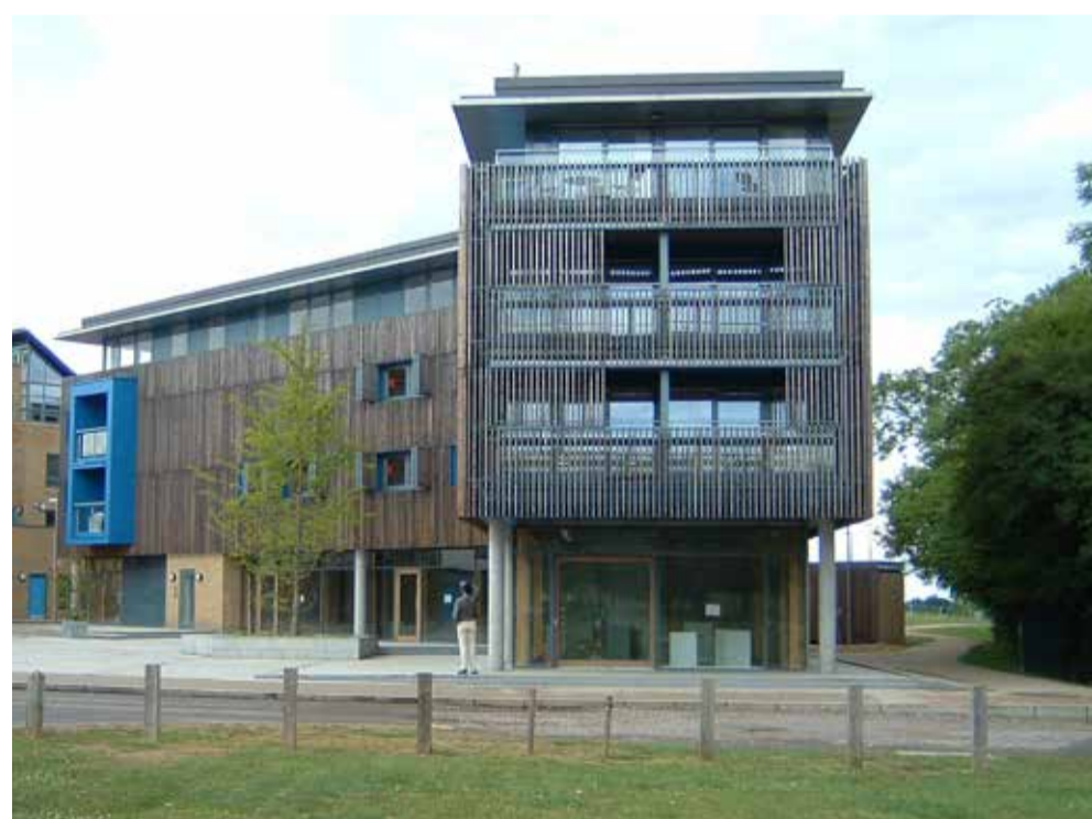
Gable end to loch: Presenting a reduced building frontage with open space in between. Upton and New Hall, Essex.
