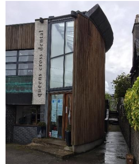
Vertical timber cladding to rear extension of Queen's Cross Dental in interesting curve design
